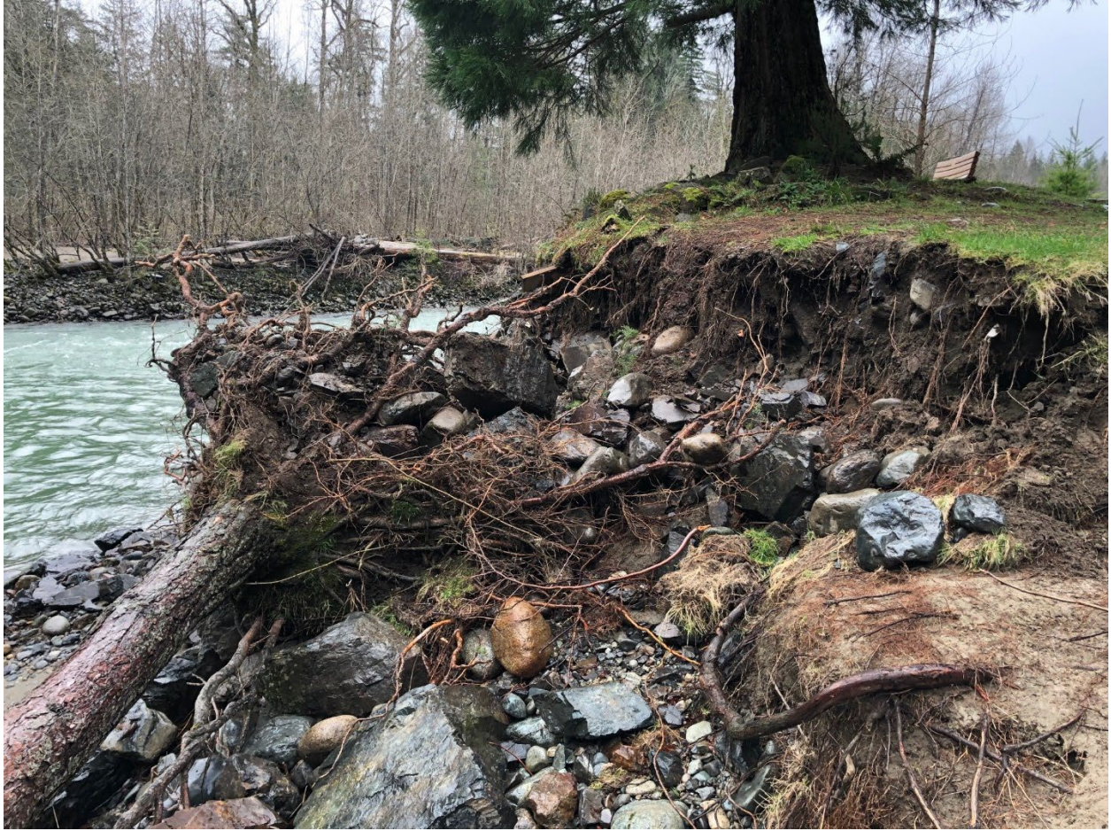
Photo 2. Damaged MTE Levee looking upstream from near the King County property line.
