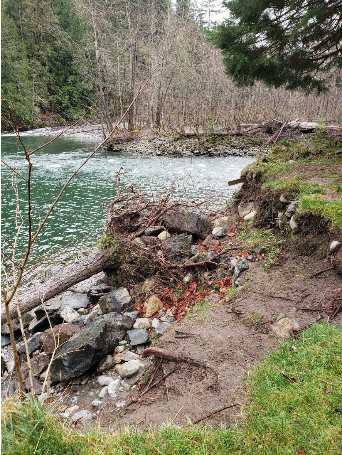
Photo 3. Alternate view of the damage to the MTE levee looking across the Middle Fork Snoqualmie River.
